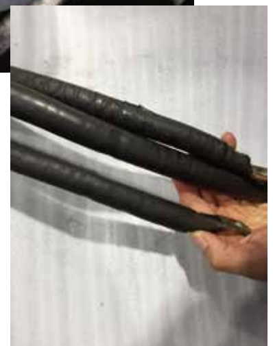
Removing wiring dirt
